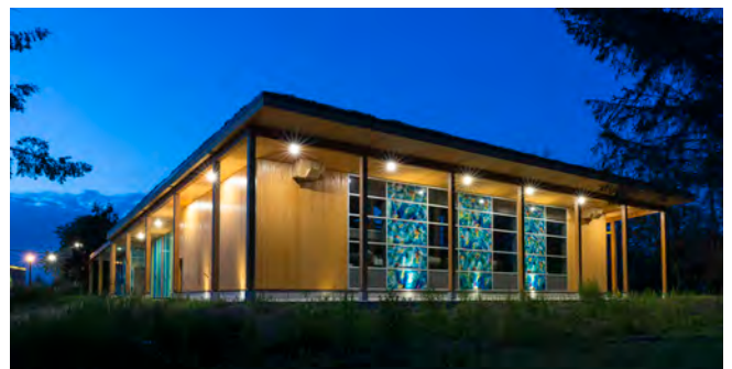
Alexandra District Energy Utility
