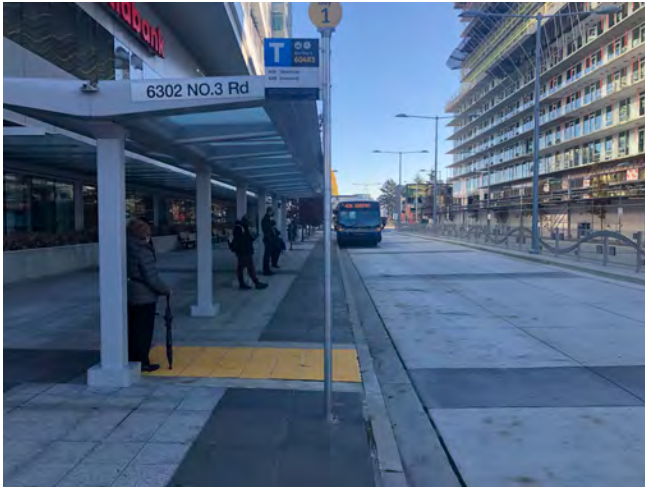
Brighthouse Off-Street Bus Exchange
