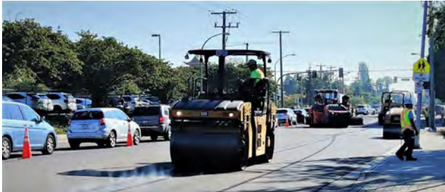
Recycled Asphalt Paving on No. 5 Road
