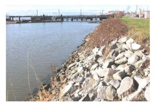
constructed or upgraded during the Fraser River Flood Control Program. Upgrades to the dikes in Steveston took place in the late 1970's. At that time, the dikes were generally upgraded with expansions to the land side and increases to crest height and width.
