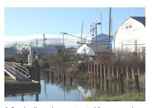
activity such as fishing or shipping. A floodwall can be constructed from a number of different materials including concrete, steel or plastic. Some floodwalls can be designed to be demountable and are only erected prior to a flood. There are some existing examples of sheet pile floodwalls in the Steveston Area.
