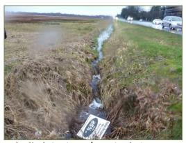
e) Headcut upstream of concrete culvert
