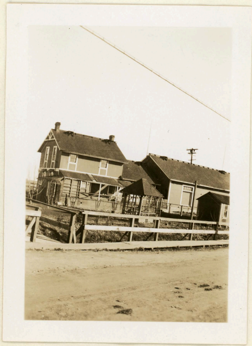
B.C. Electric Station Steveston
