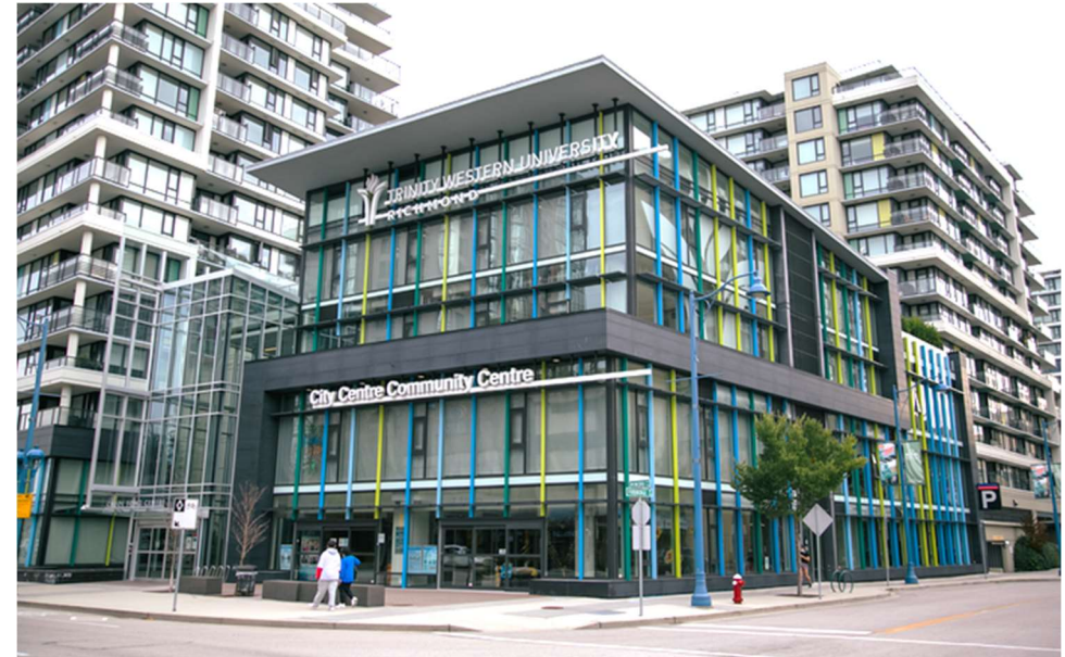
Accessible Route Highlighted by Paving Contrast.
