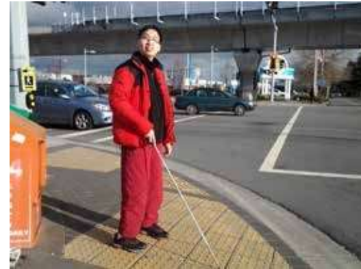
Barrier-free design incorporates a clear accessible path with cane detectability and high colour contrast.
