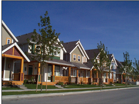
Townhouses with Front Doors Visible and Accessible from the Road
